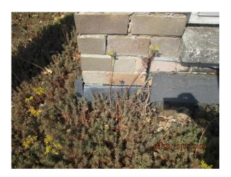
Plant growth and cracking to brickwork, pitched roof 2
