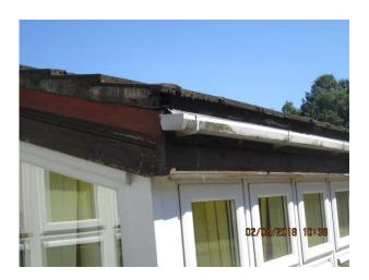
Pitched roof 5 – raised tiles and infill barge board strip
