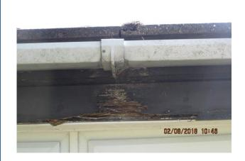
Leaking gutter water damage to fascia
