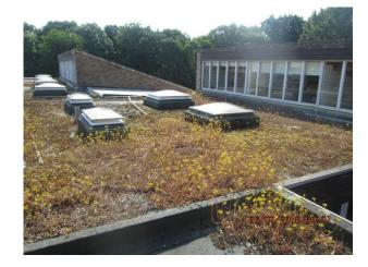
Main roof – plant growth. Pitched roof 4 on right and pitched roof 5 on left
