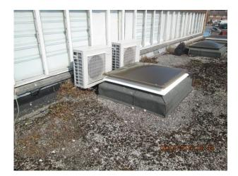
Main roof – Rooflight and Air conditioning condenser on asphalt roof adjacent to pitched roof 3
