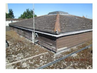
Hall roof. Decaying cladding and poor guttering
