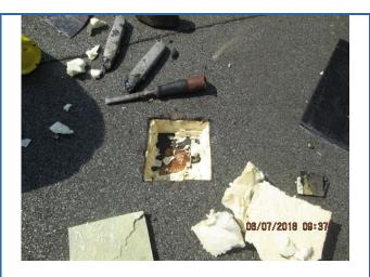
Core Sample of small felt roof 1
