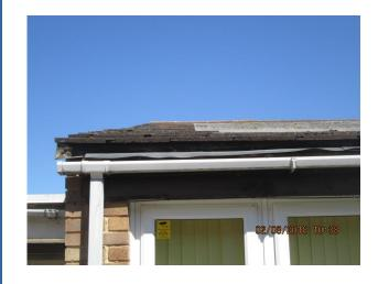
Pitched roof 5 – raised tiles but gutter at original lower level
