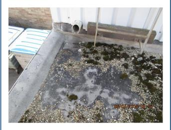
Gutter outlet of tank room roof onto main roof
