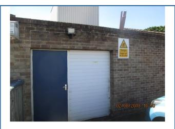
Lintol rusting and lifting brickwork over store door
