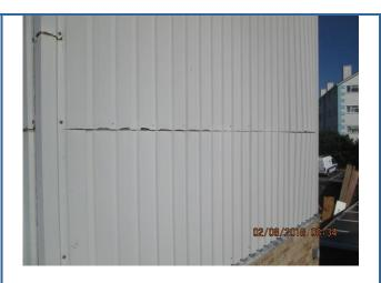
Bulge in cladding – East elevation
