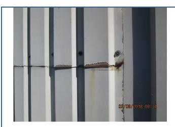
Corroding Tank room cladding at sheet ends
