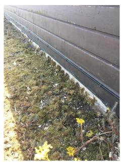
The cladding will need to be raised to allow the introduction of insulation onto this roof.
