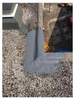
This picture shows where the detailing is failing and water ingress has occurred.
