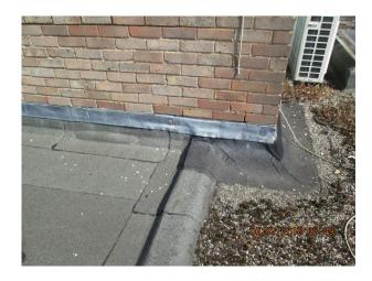
Small felt roof 1 – upstand, flashings screw fixed and blister
