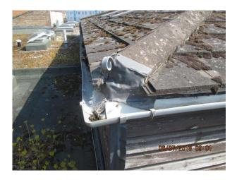
Patch repair to hall roof hip tiles
