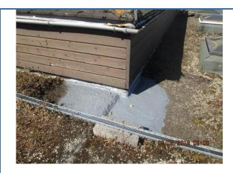
Recent Acrypol repair to asphalt roof adjacent to hall roof North East corner
