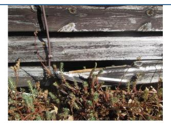
Broken hall roof cladding and plant growth below
