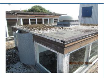
Raised kitchen roof – asphalt with patch repairs
