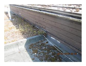
Small felt roof 2 to lower level showing step down from main roof
