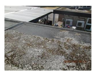
Patch repair to main asphalt roof adjacent small roof 3
