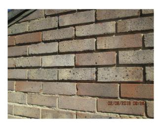
Pitched roof 2 – eroded pointing
