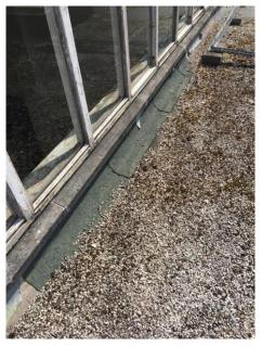
The area under the windows shows where the cover flashing is missing and a repair using felt has been carried out.
