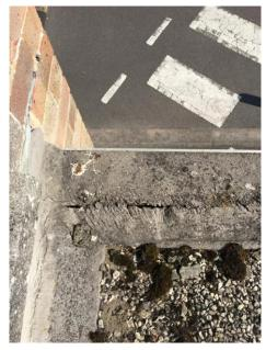
There are splits and cracks in the asphalt. This school was built in 1974 and this is probably the original roof.
