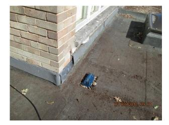
Felt roof 2 swept off exposing felt and gully
