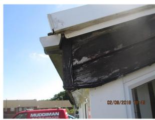
Degraded timber barge board
