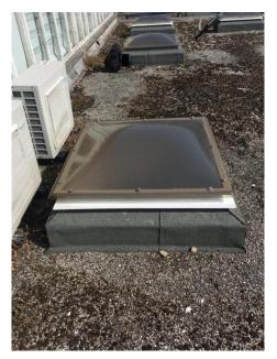
All the roof lights will be changed in the event of a complete refurbishment. The new lights will be triple skinned poly carbonate.
