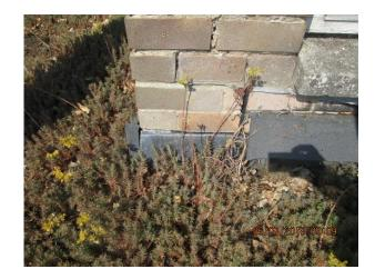
Brickwork cracking and excessive plant growth on roof
