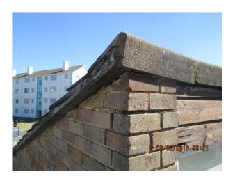
Pitched roof 1, lifting and opening mortar joints
