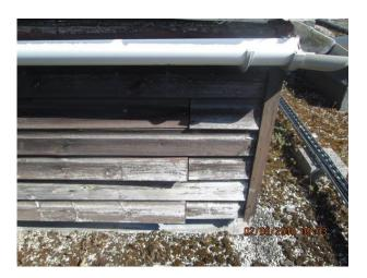
Warped and cracked cladding
