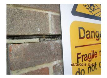
Rusting lintol lifting brickwork
