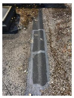
Many areas of this roof have been repaired using either Aquapol or a commodity membrane.
