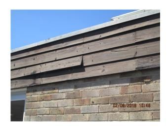
Example of warped and cracking fascia with minimal decoration
