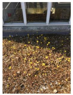
With the introduction of insulation on this roof the windows will need to be raised.
